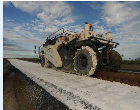
Camp Cable Road intersection on the Mount Lindsay Highway: Foam bitumen base successfully withstood inundation on the existing pavement and widened sections
