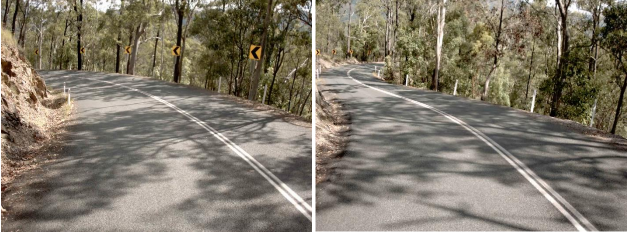
Figure B.2: Rural Road 2 – 2025
