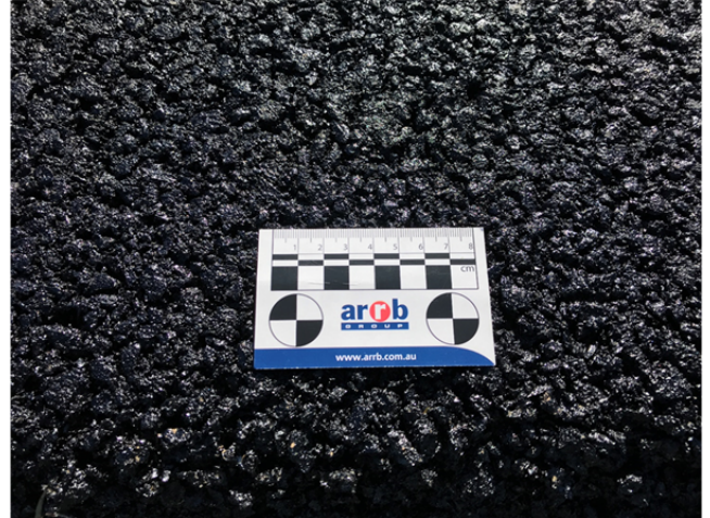
Finished crumb rubber modified gap graded asphalt surface
