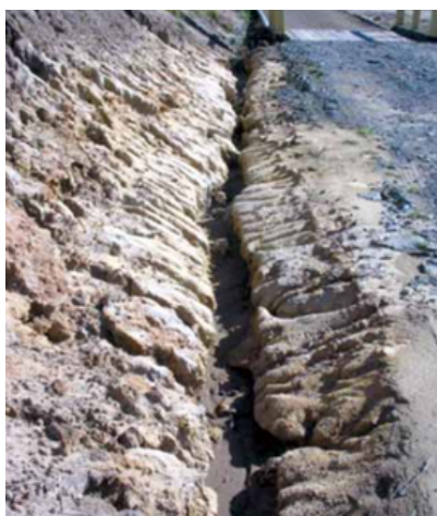
Figure 2.5: Example of table drain constructed in dispersive soils – Source: Hardie et al. (2009)
