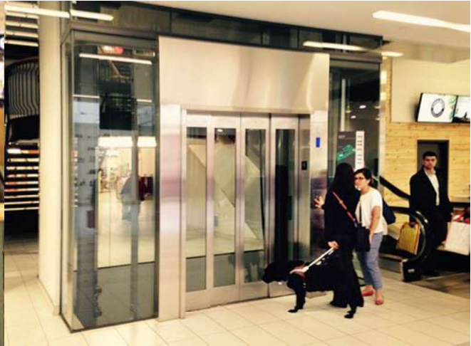
Figure 3.4 After refurbishment. Panoramic lift at west end that fits three wheelchairs
