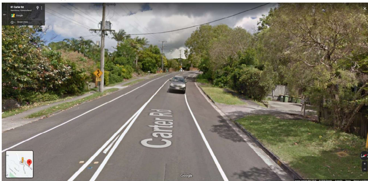
Figure 6.8 South-east from 81 Carter Rd, Nambour – visual representation of where the end of the slope is not apparent
