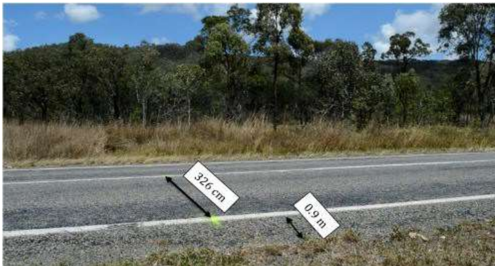
Fig. 26. Roadside Conditions for Site 1
