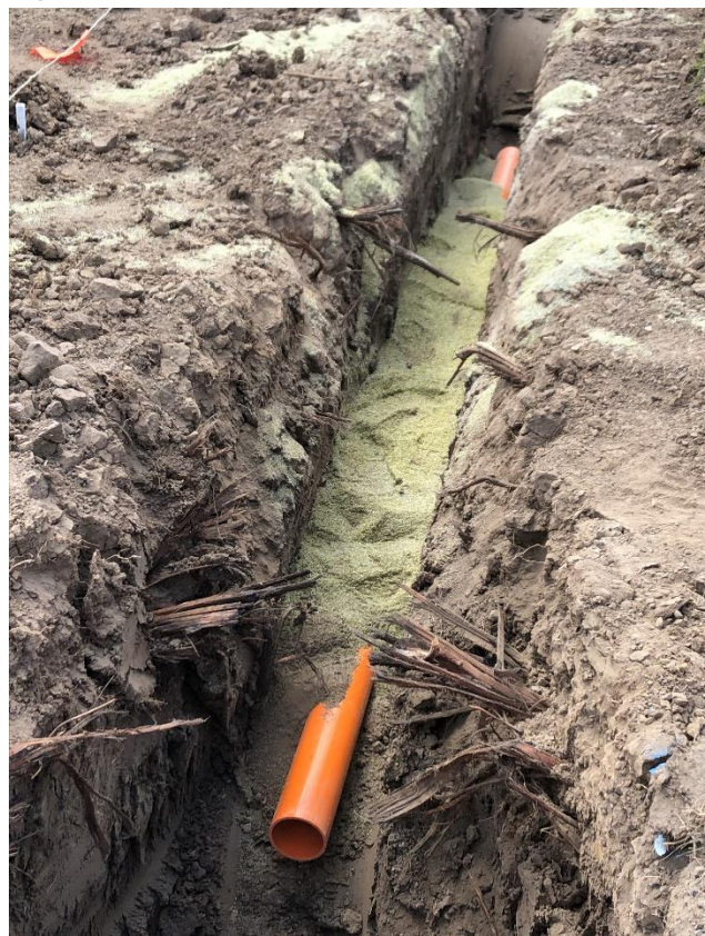
Figure 4.2: RCG over conduit pipe
