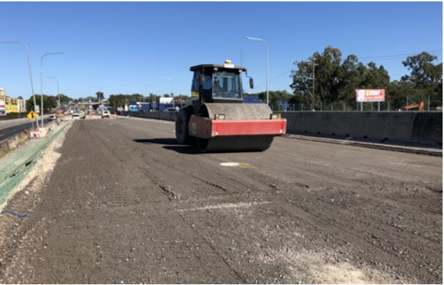
Intelligent Compaction fieldwork demonstration in Queensland. Image Source: NACOE (2020)
