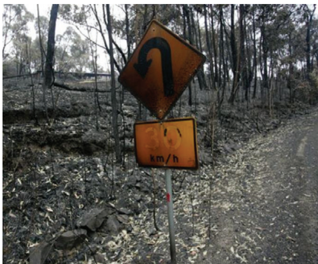
Image: Bushfire damage to safety infrastructure Source: Mancini (2020)
