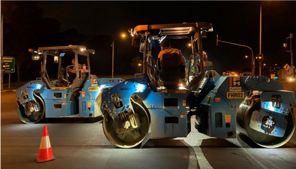
Figure 1.1: Intelligent compaction rollers – asphalt work
