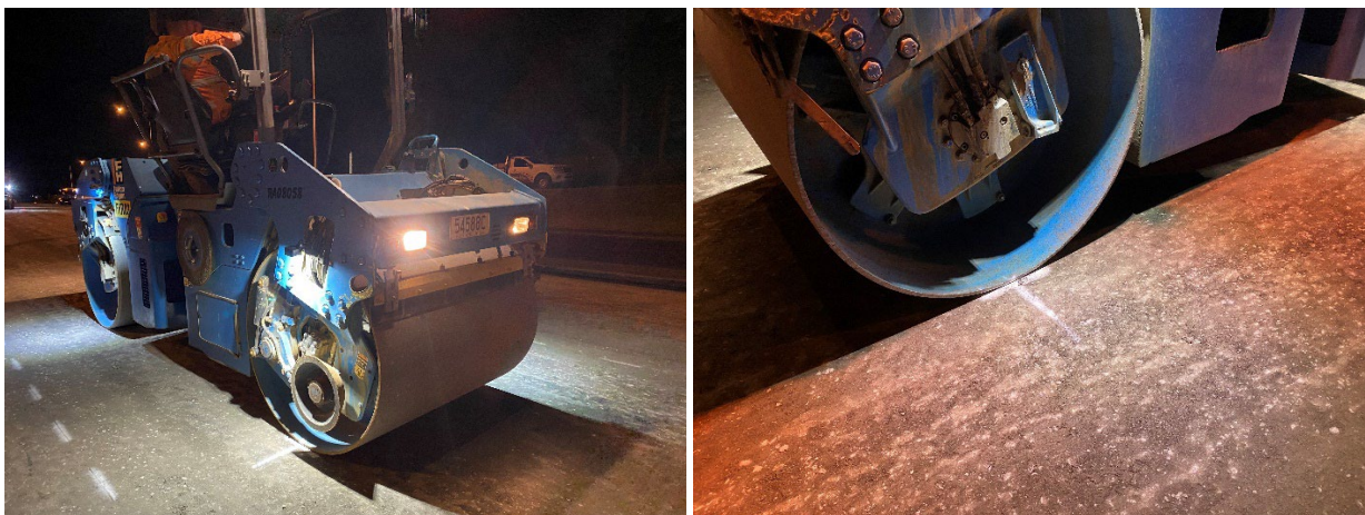
Figure 2.14: GPS verification – marking the drum edges
