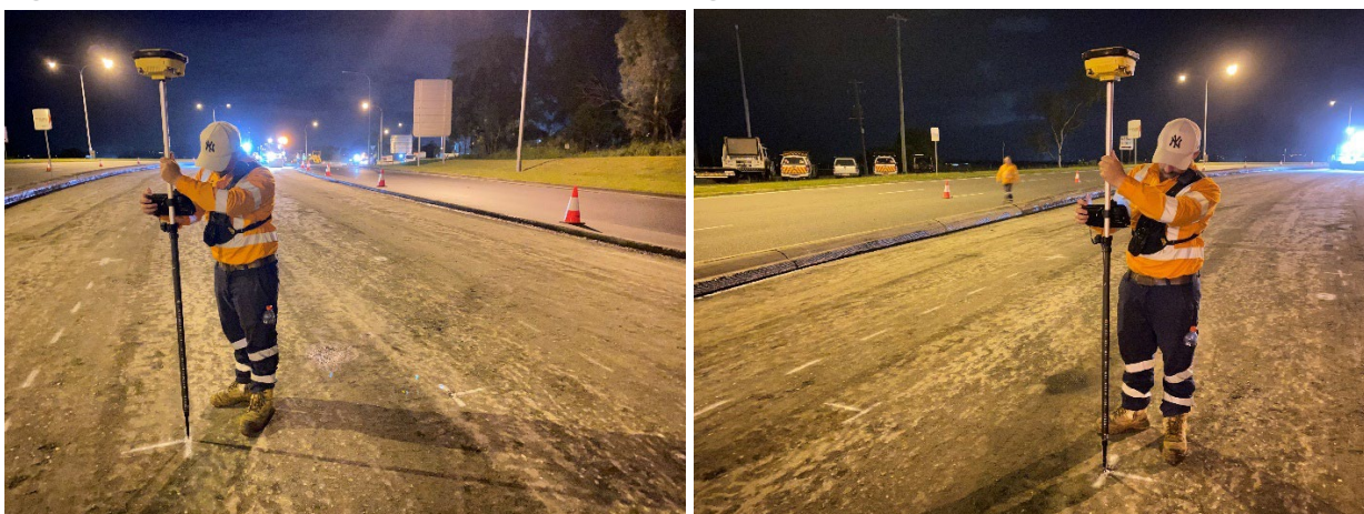
Figure 2.15: GPS verification – coordinates of drum edges
